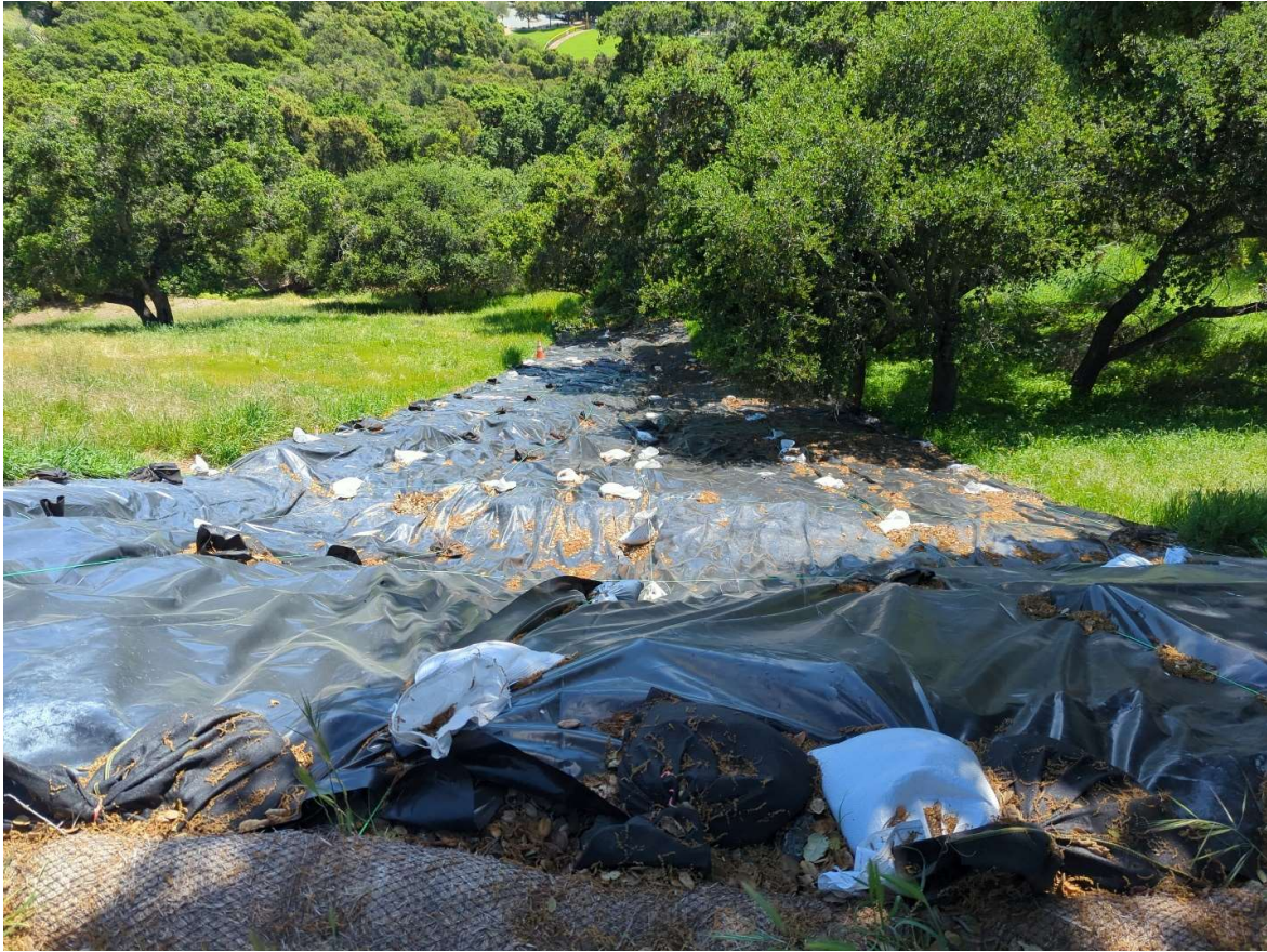
Exhibit 2. Temporarily stabilized landslide from the 2022-2023 storms along Dartmouth Ave above Arguello Park. Photo taken by WRA 4/12/24.
